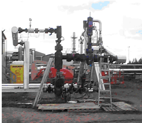
Photograph Copyright Sealweld Corporation
