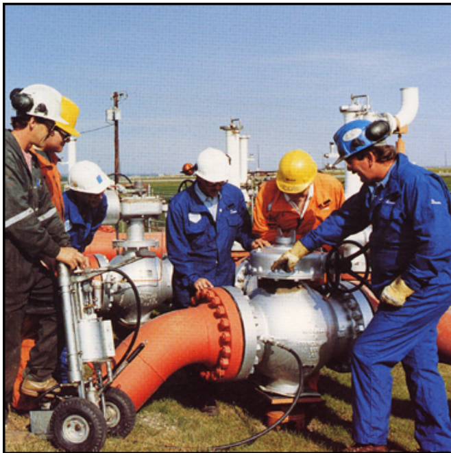
Sealweld® On-site Training
