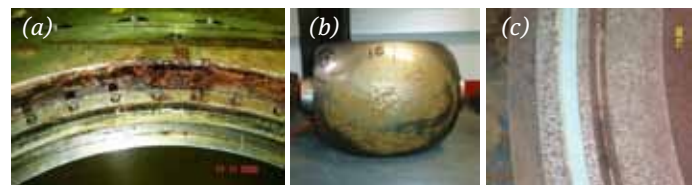
Figure 7: Examples of damage due to improper test fluid control: (a) a severe corrosion attack at the seat pocket area; (b) galvanic corrosion due to testing by untreated seawater; and (c) pitting corrosion in a 56 inch diameter ball valve, which was tested using water with a high chloride content.
