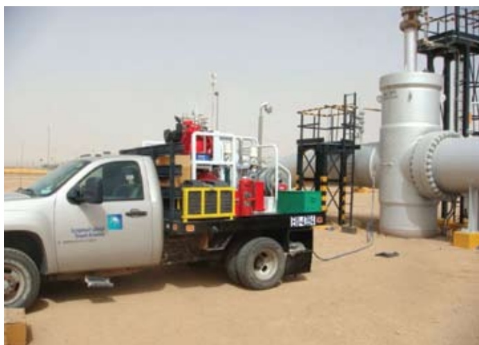
'Figure 5: Repair internal passing of 56" through conduit gate valve.'
