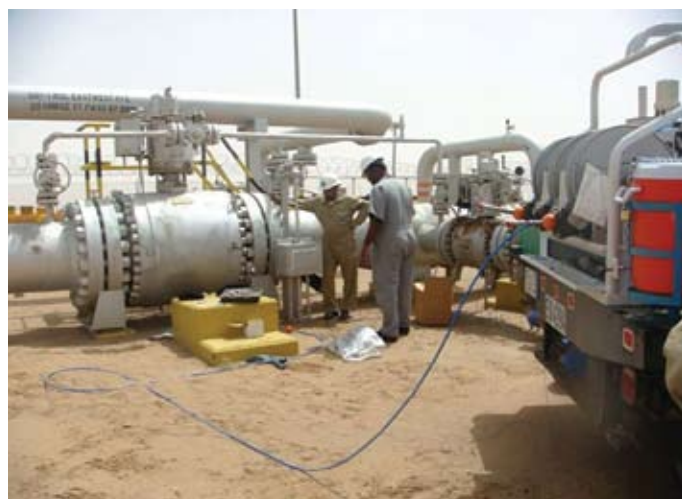
'Figure 6: Repair internal passing of 36" Ball Valve.'
